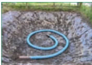
The outlet in the base of the pit is fitted with a coil of 100mm diameter perforated drainage pipe. Pumps are fitted to the inlet and outlets.
