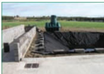
The pit for the biobed is lined with a geotextile membrane followed by a 1.5mm thick, one-piece liner of a type suitable for a small reservoir.
