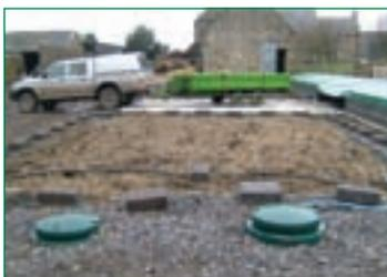
The drip irrigation system feeds the liquid into the top of the biobed. It trickles through the biomix and emerges as clean water.
