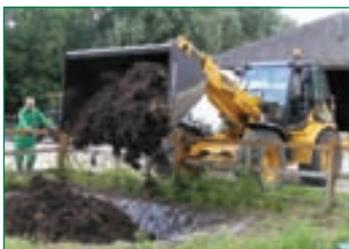
The biomix is then filled into the pit and left to settle and turfed over. The grass needs to establish before the biobed is used. The biomix lasts five years.
