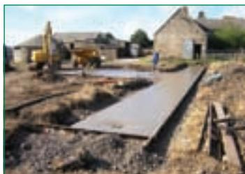
The top of the concrete 'T' allows the boom to be opened so that tank washings can be sprayed out, collected and diverted to the biobed.
