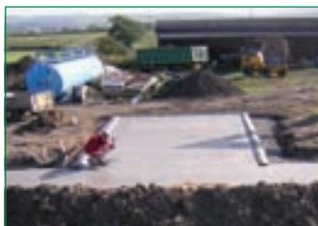
The concrete filling area takes shape, with the 300mm wide by 100mm high bunding on the edges to contain spills. The pad slopes towards the drain.
